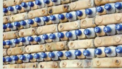
Stacked into a wall, used, sand-filled plastic water bottles get a second life.
