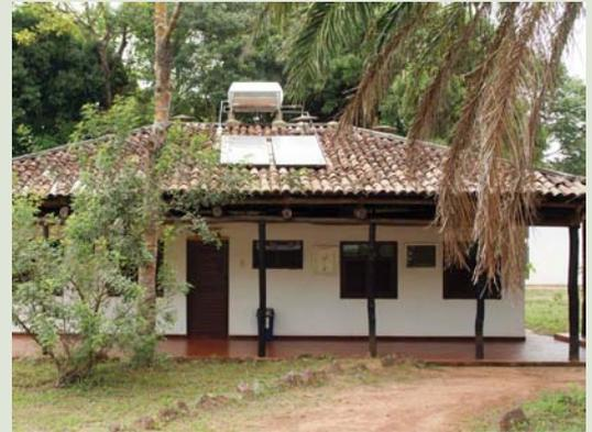
The Gaviotans' multiuse meeting hall (left) and this traditional house (above) are constructed of hand-pressed, earthen-cement bricks.
